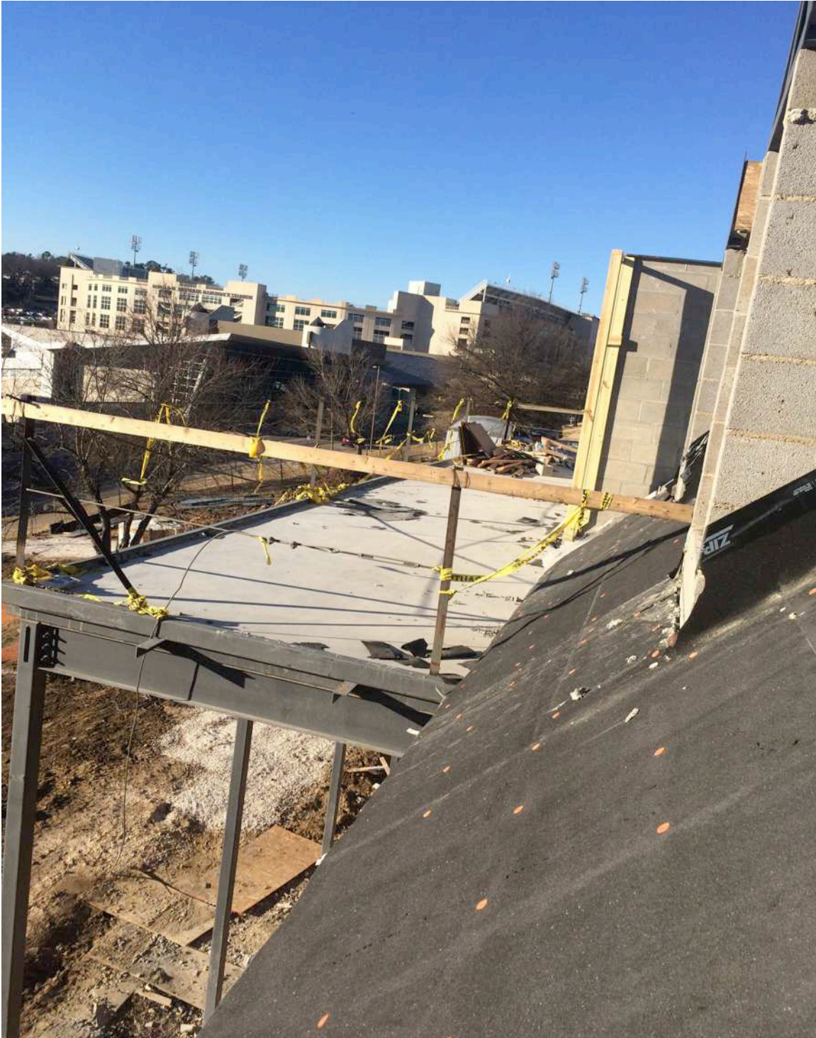
View of the renovated balcony.
